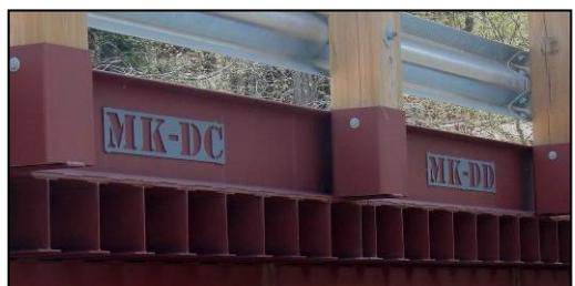
Once the substructure has been completed, connect the diaphragms (hand tight - to allow some movement) to the interior stringer(s) using the structural bolts provided and lift and place the stringer(s) into position. Block/brace the interior stringer(s) and then lift and place each of the exterior stringers. Connect the end diaphragms (hand tight - to allow some movement) at each end between the interior and exterior stringers.
